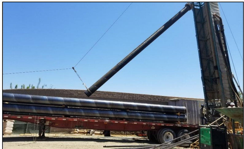
Grand Avenue Well Drilling Activities
